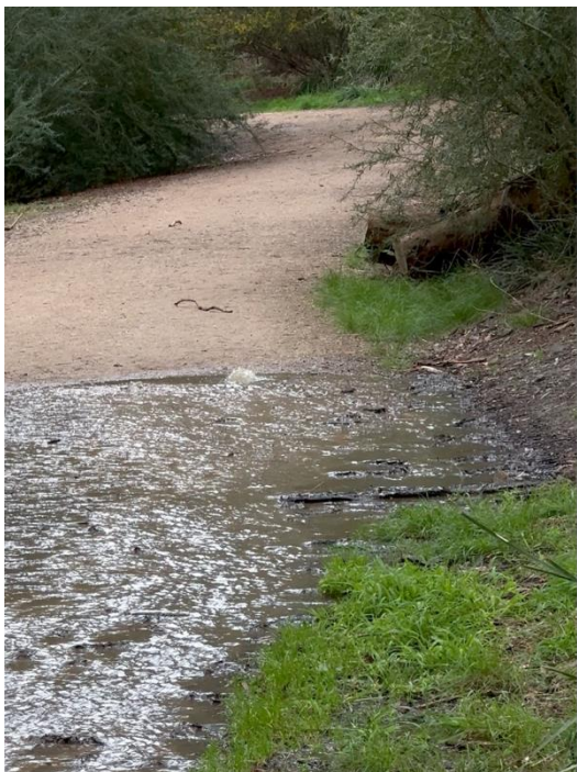
Sewerage leak near Stephensons Road entrance on 30 August
